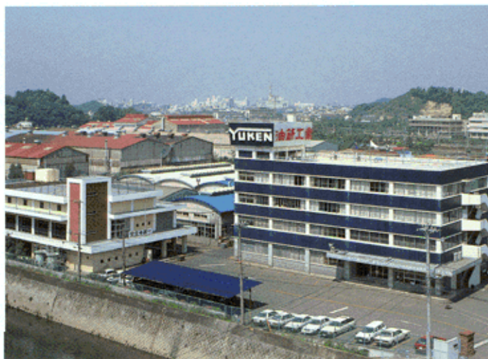
Head Office & Fujisawa Factory
