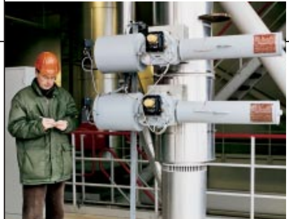
Bettis actuators in service at a major coal gasification plant
